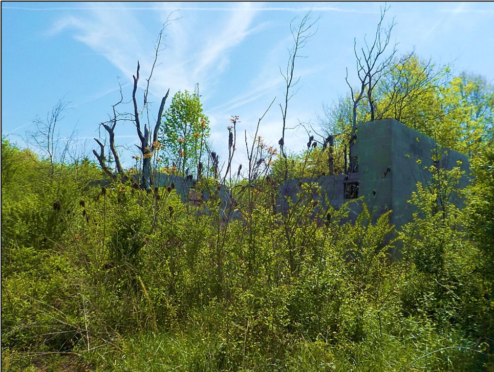
Figure 13. Structure indicated on the 1957 and 1983 Fountain Inn topographic maps.
