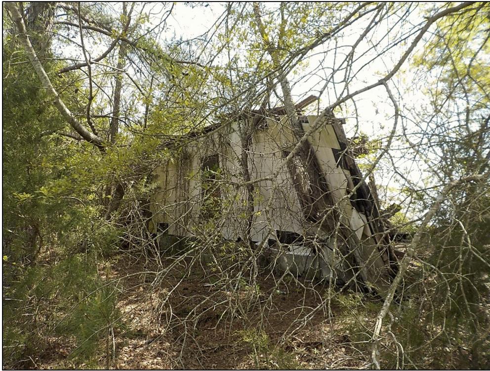
Figure 14. Structure indicated on the 1957 and 1983 Fountain Inn topographic maps.
